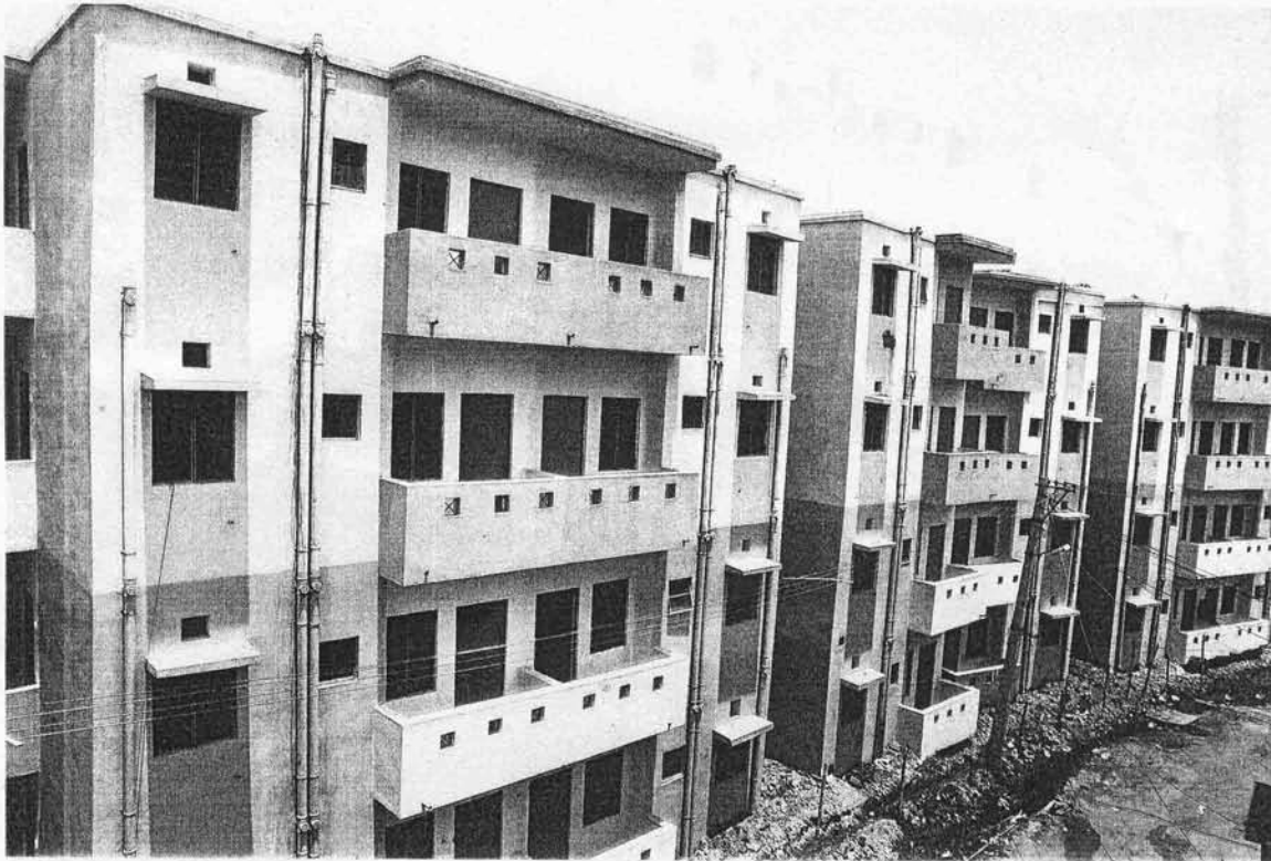
Side view of BSUP units at Isopur
