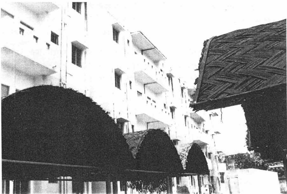
View of the vending zone in the back ground of BSUP units at Isopur
