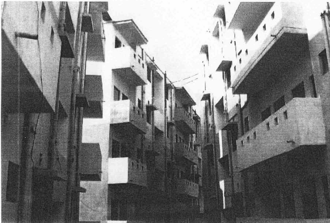
Over all view of the internal Building Blocks at Isopur
